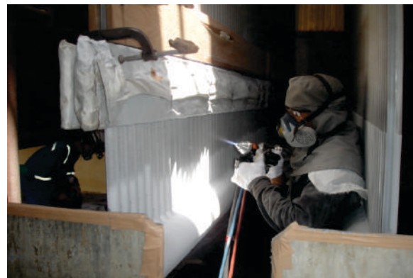
Aluminum Coating on ORV Panel
