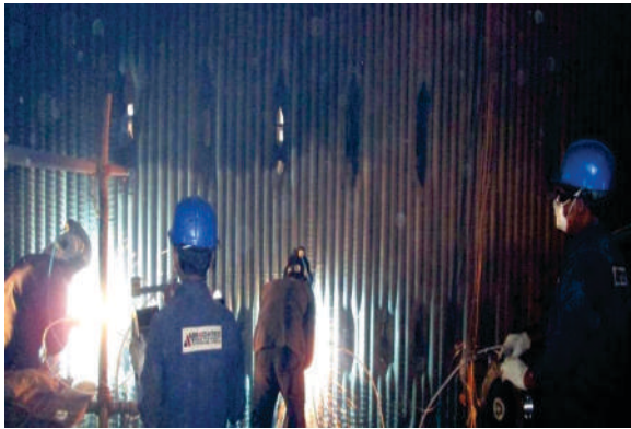
ARC Spray Coating on Recovery Boiler
