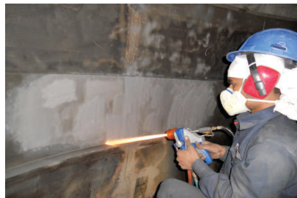
In-Situ HVOF Coating on Pivot Ring
