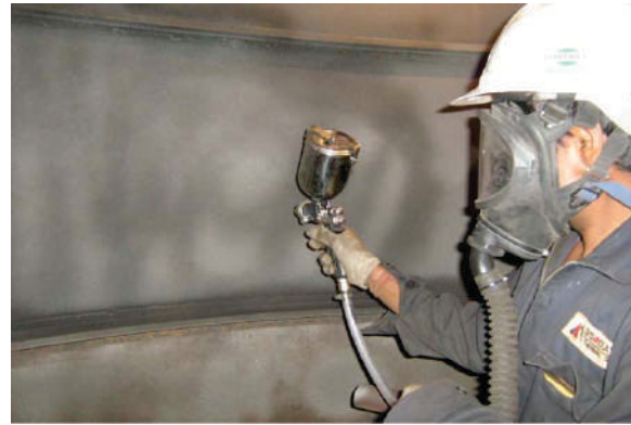
Sealant Application inside Coloumn
