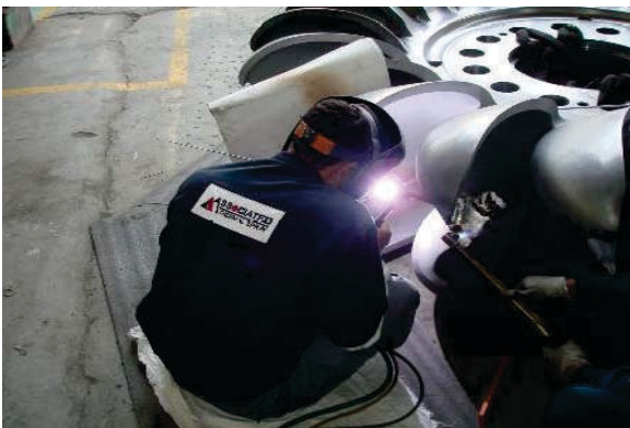
Weld Repair of Pelton Bucket
